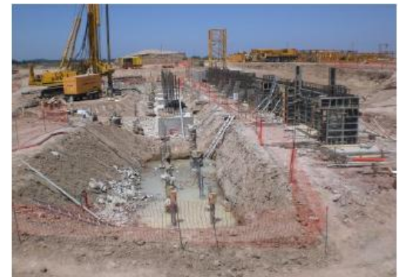
Recovery boiler: Pile caps zone
