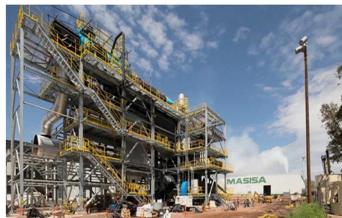
Biomass Plant, Durango
